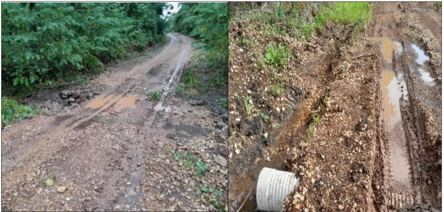
FIGURES 82-83. CROSSINGS AND EXTERNAL ROAD REHABILITATION TOWARDS THE FARMS LASTENIA.
